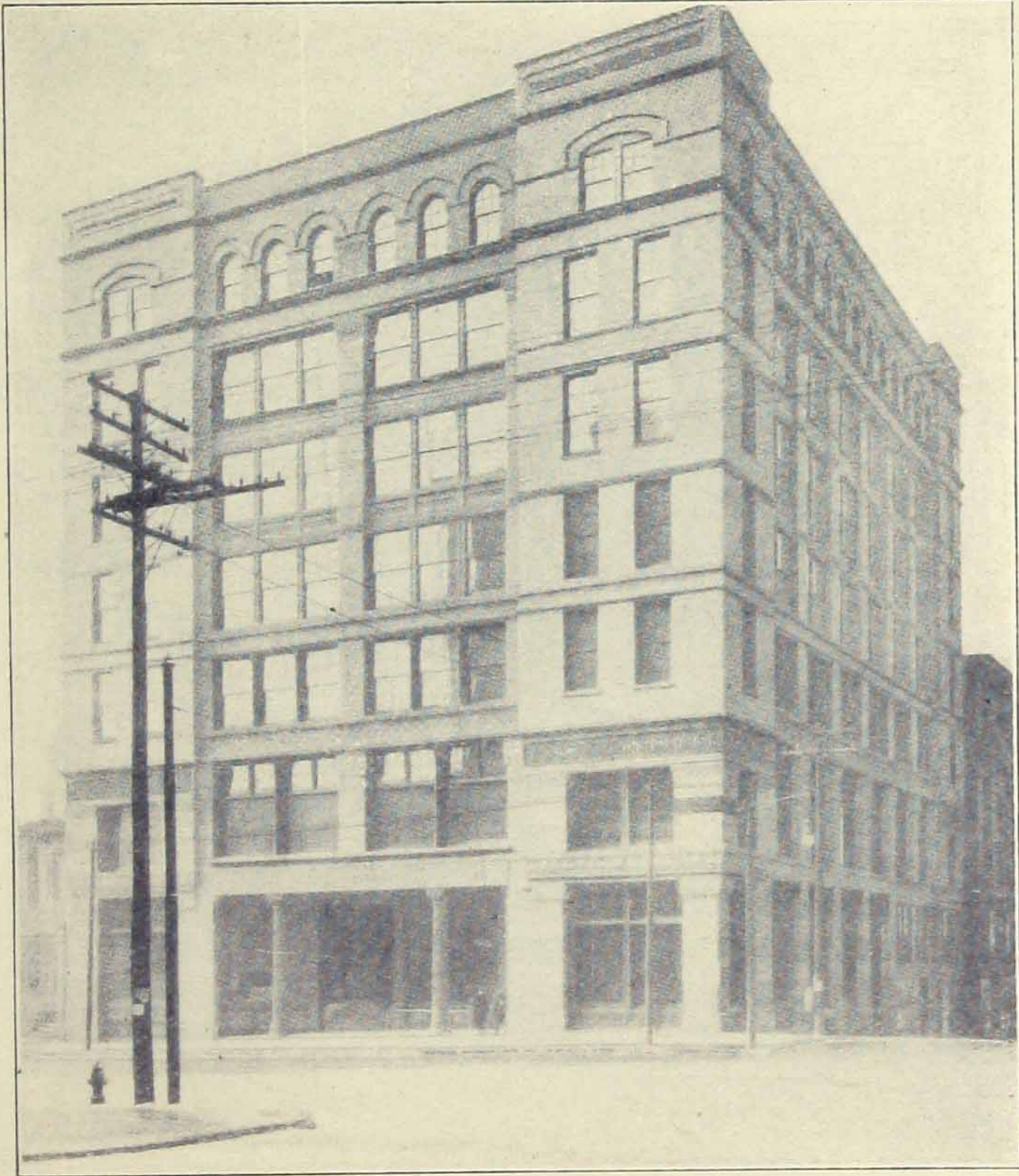
THE REMODELED BRYANT BUILDING, KANSAS CITY, MO.
